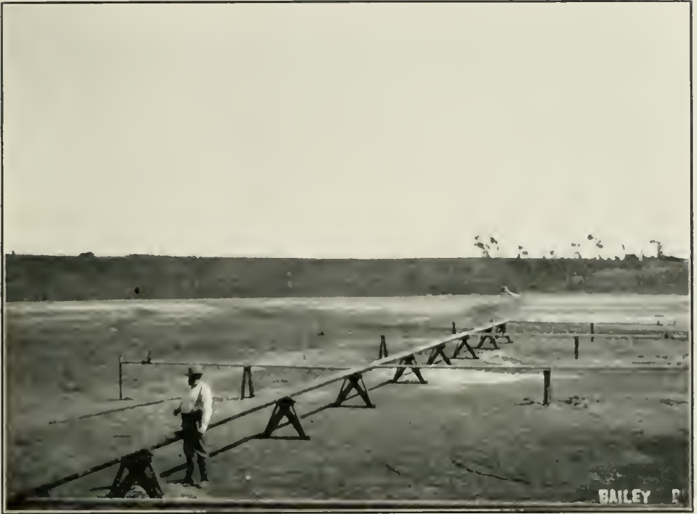
SALT WORKS NEAR OCEANSIDE, SAN DIEGO COUNTY. SIX 50-FOOT WELLS CONNECTED WITH ONE PUMP FOR DRAWING BRINE FROM THE LAGOON TO THE VATS.
